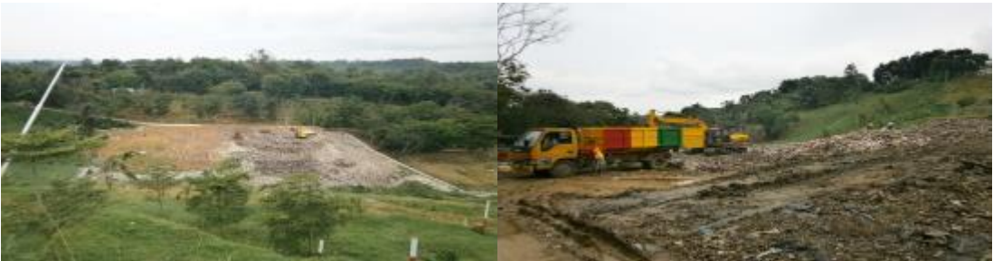
Figure 5-4 Pictures of Tenggara landfill
