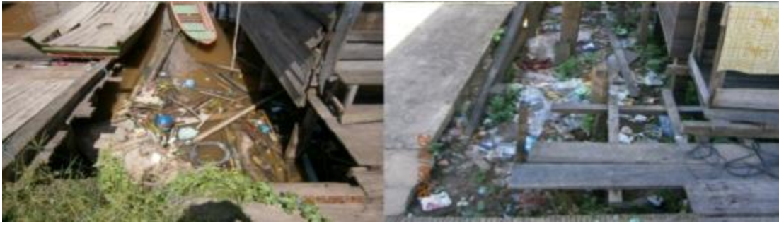
Figure A-2 waste accumulation in the Mahakam river and under housing in Muara Kaman subdistrict
