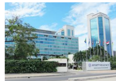
Figure 116. Hyatt Regency Dar es Salaam, The Kilimanjaro.
