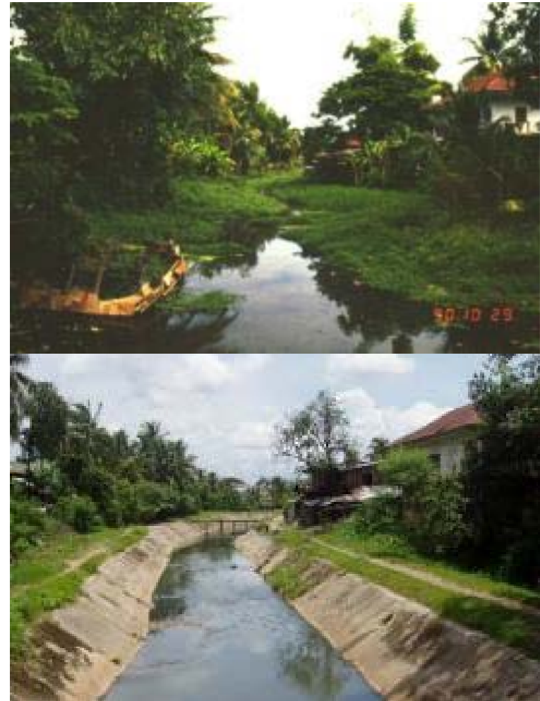
Fig. 2 The Hong Ke, part of the natural drainage network of Vientiane, in 1990 and in 2003 after rectification.
