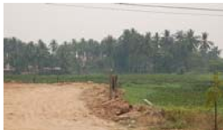
Filling of the wetland to make place for new settlements.
