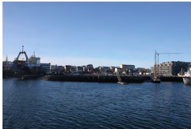
186 - The harbour work has developed from the human hand to machines.
