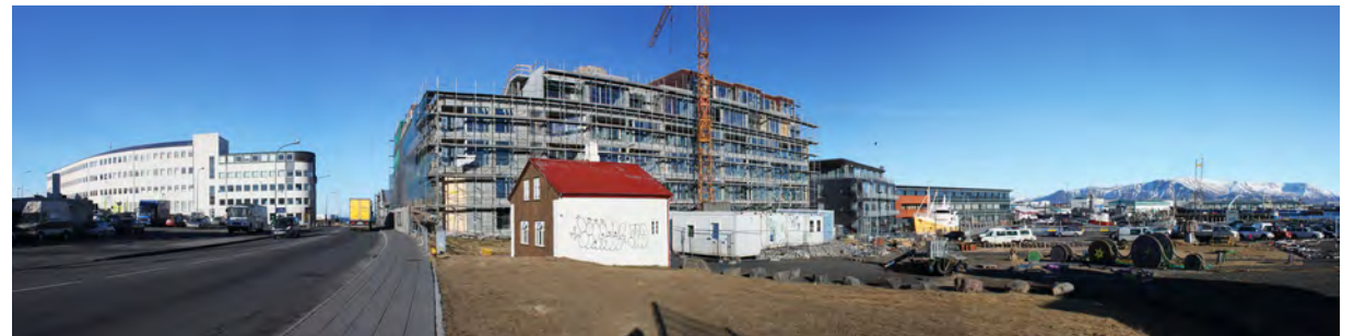
285 - Lot number 02 according the Municipal plan. The Residential house does not harmonize at all with the preserved stone house.
