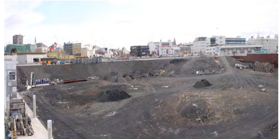
156 - The constructions have already begun.
