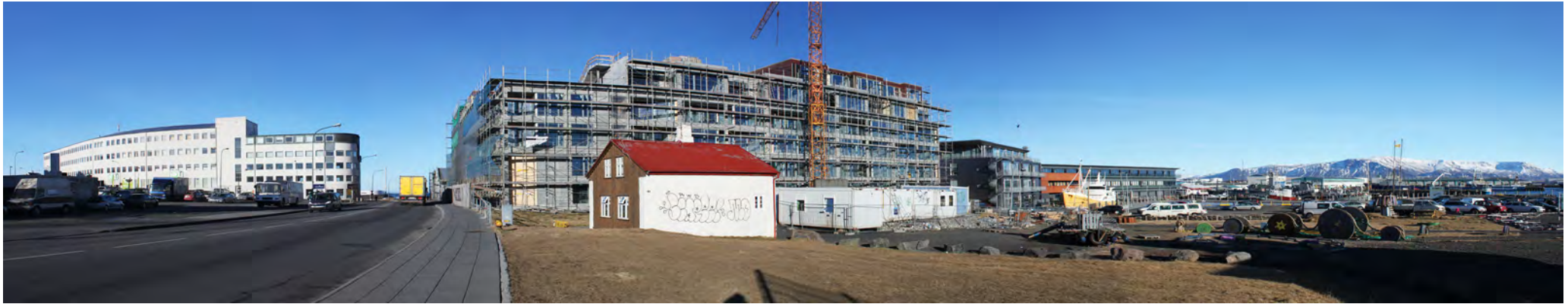
266 - The pre-existing buildings in the harbour area vary in scale.
