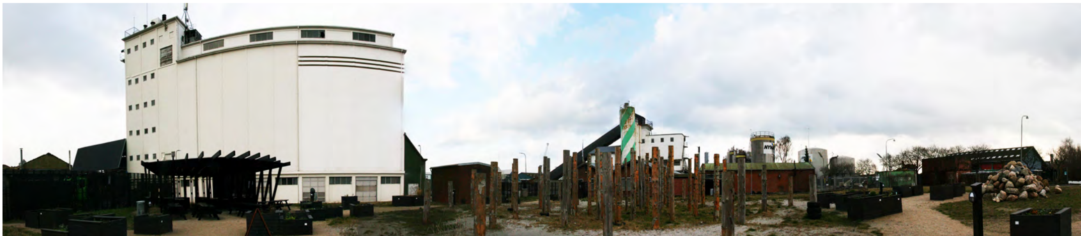
59 - The main materials are; concrete and bare brick houses, containers and small wooden huts, high corrugated iron tanks, big rock hillocks, steel and piers.
