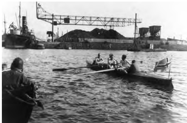
137 - After the improvement of the piers began, bigger ships were able to land at the harbour site.
