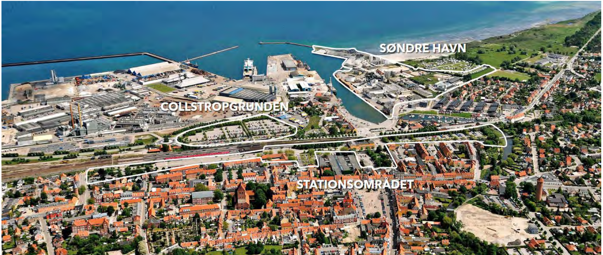
17- Aerial image of the three construction areas. This thesis focuses on the South harbour area.
