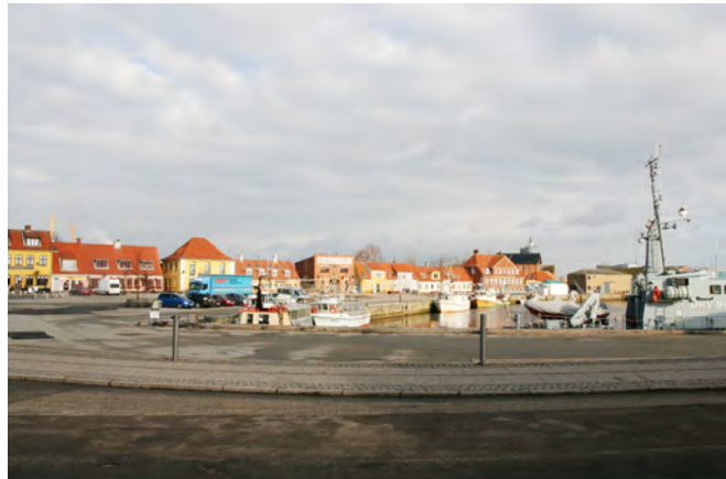
26 The main building materials are brick, concrete and stone.
