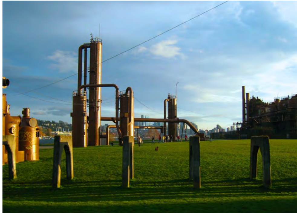
Figure 22. Industrail elements from the previous time when the industry was in use have been preserved. Photo: © "064 of 365 - Gas Works Park" by Yogesh Mhatre (CC BY 2.0)
