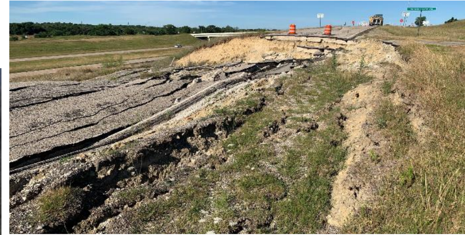
Service Road along US 75
