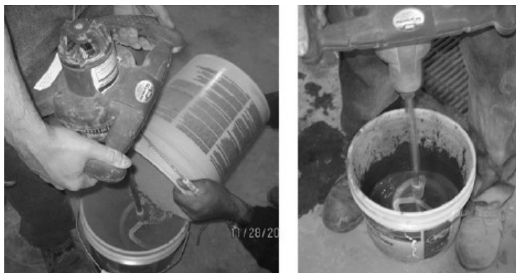
Figure 3. 47 - Mixing procedure (Contractor Training Manual)
