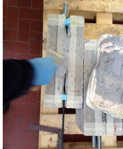
Figure 4. 7 – Placement of thixotropic resin in the groove
