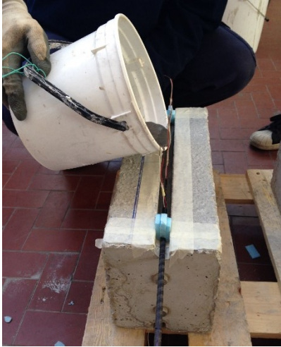
Figure 4. 6 – Casting of cementitious mortar in the groove
