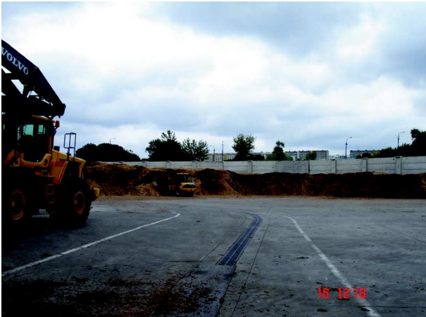
Figure 5. The storage yard for the biomass fed into the system supplying the power block.
