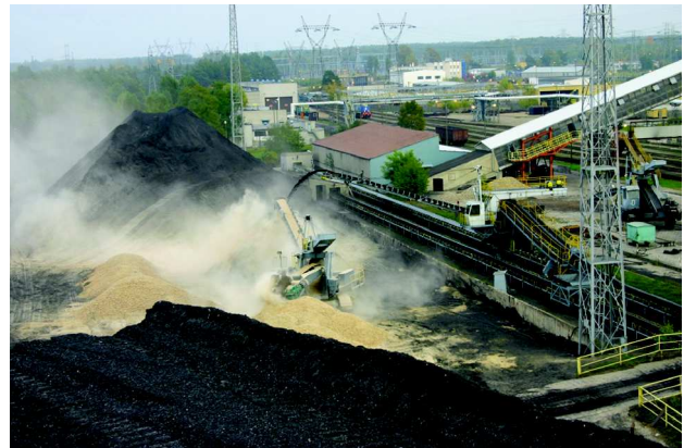
Figure 9. The storage yard for the coal and biomass for the production of the coal and biomass mixture for the cogeneration process
