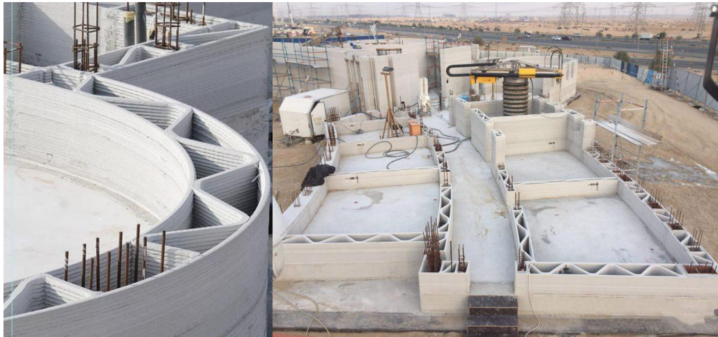
Figure 1: World's largest 3D concrete printed building in Dubai (Apis-Cor built the office with a robotic printer, 2020 [14])
