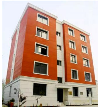
Figure 3. Winsun 6-Story tall 3D printed building
