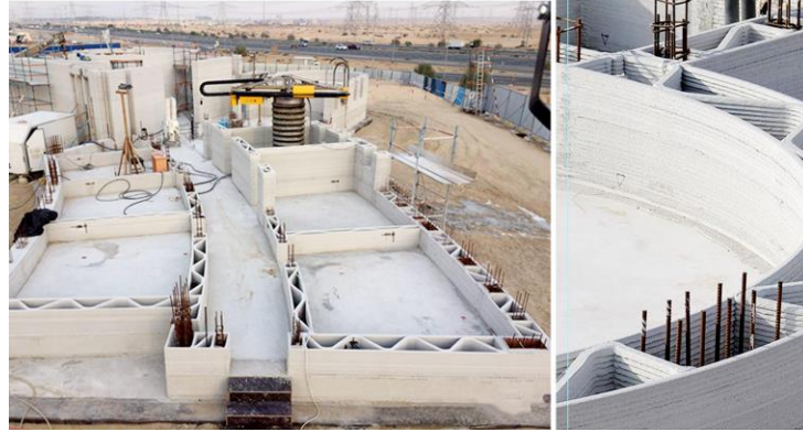
Figure 2. One can see reinforcement embedded conventionally in Dubai Municipality Building
