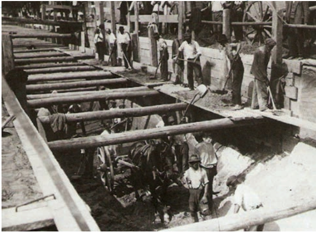
Figure 9: The work ditch which was fitted for the horse-drawn carriage in 1910 (Juhász, 2008).
