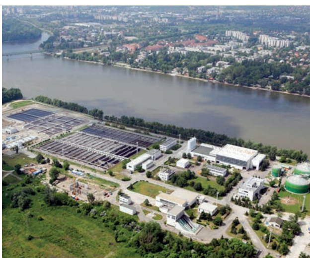
Figure 20: North-pest WWTP in 2010 (Brochure).
