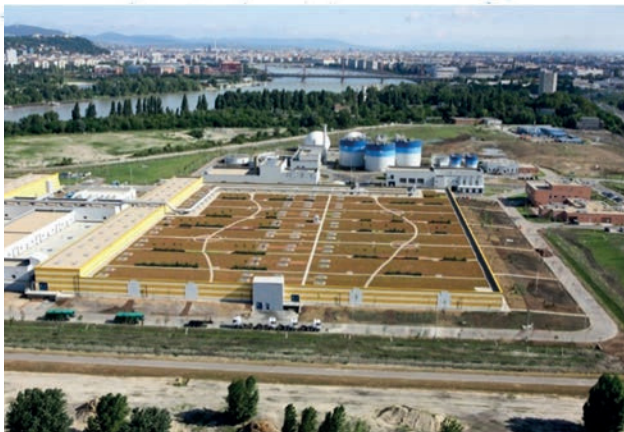
Figure 22: The covered Budapest Central WWTP in 2010 (Brochure).
