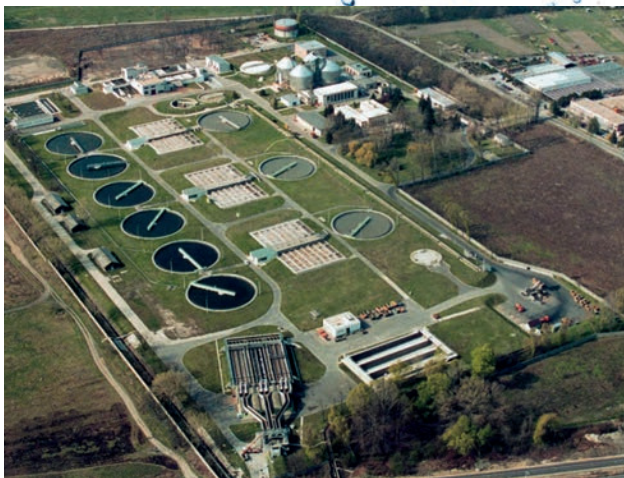
Figure 19: South-pest WWTP in 2003 (Brochure).
