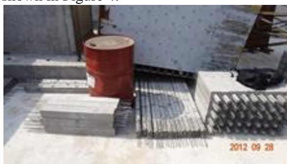
Figure 4. Precast elements on site
