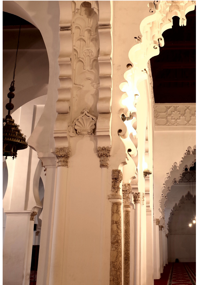
Figure 9. Columns and capitals attached to the jamb of the access arch to the maqşūra area in the central nave of the second phase of the Kutubiyya mosque. The one on the right is rather smaller, perhaps due to the existence of the groove for the screen of the enclosure that has been probably hidden. Author: A. Almagro.
