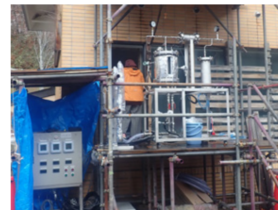
Fig.3 Large type demonstration test equipment for hydrogen generation.
