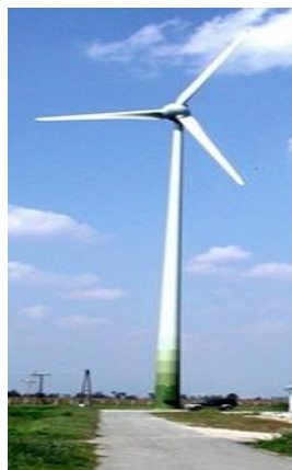
Illustration 2. The first wind power connected to the Hungarian electricity network (Kulcs, 2002) [19]
