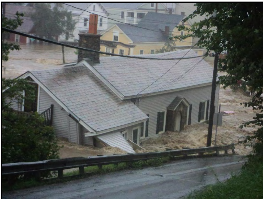
Wilmington, VT after Tropical Storm Irene in 2011. Photo by Eric Craven 8/28/11. Used with permission.
