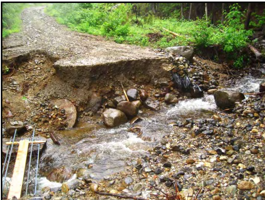
NH residents used a foot bridge for several weeks to access their home after an extreme precipitation event destroyed the road.
