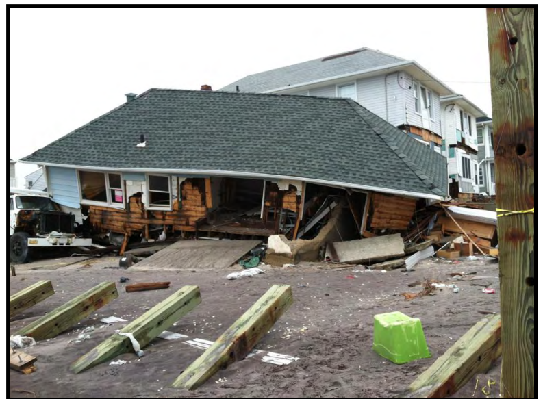
Rockaways, New York, after Hurricane Sandy. Photo by Mary McKenna.
