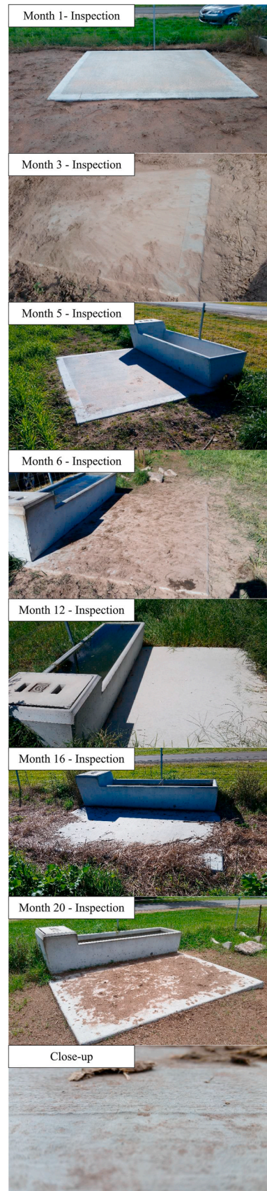
Fig. 9. 15% CO 2 Concrete slab 2 visual inspections.
