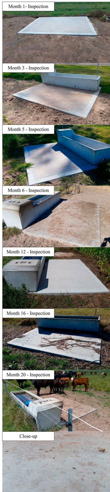
Fig. 8. 15% CO 2 concrete slab 1 visual inspections.
