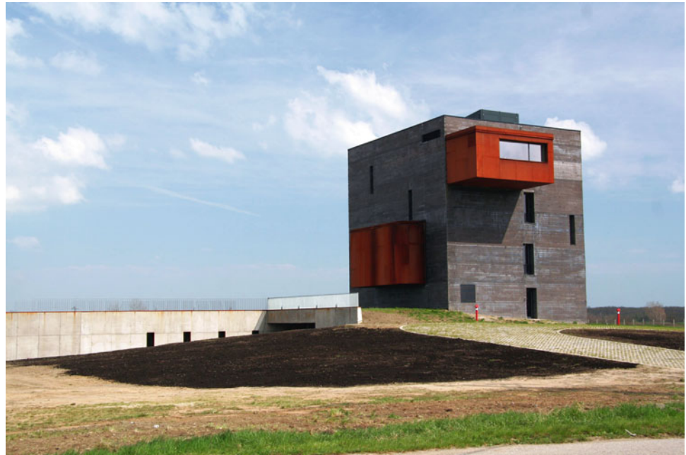
Fig. 7.10 The Volcano House at the foot of the Ság hill provides an instructive insight into the nature of volcanic processes. Photo Szabolcs Harangi
