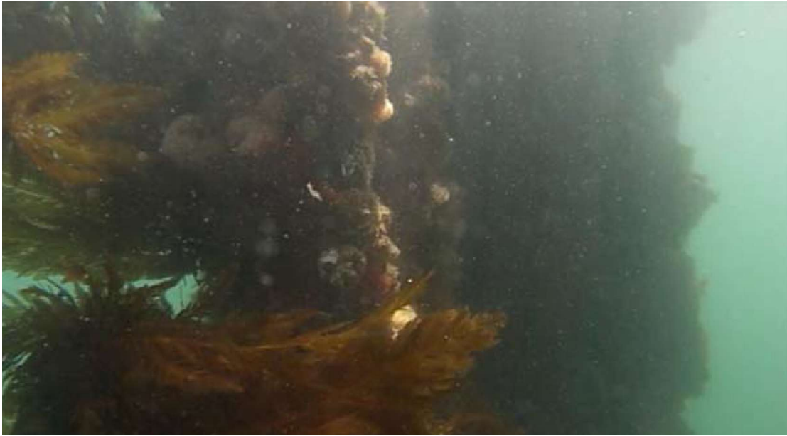
Figure 5. Underwater sea life growth on I-beam track after six months (Balingit, Spieler, & Jen, 2013).
