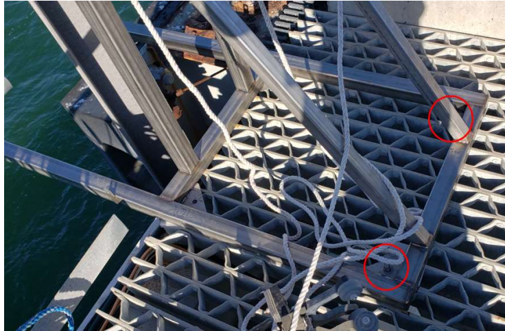
Figure 47. Assembly is bolted down to pier deck using J-bolts.
