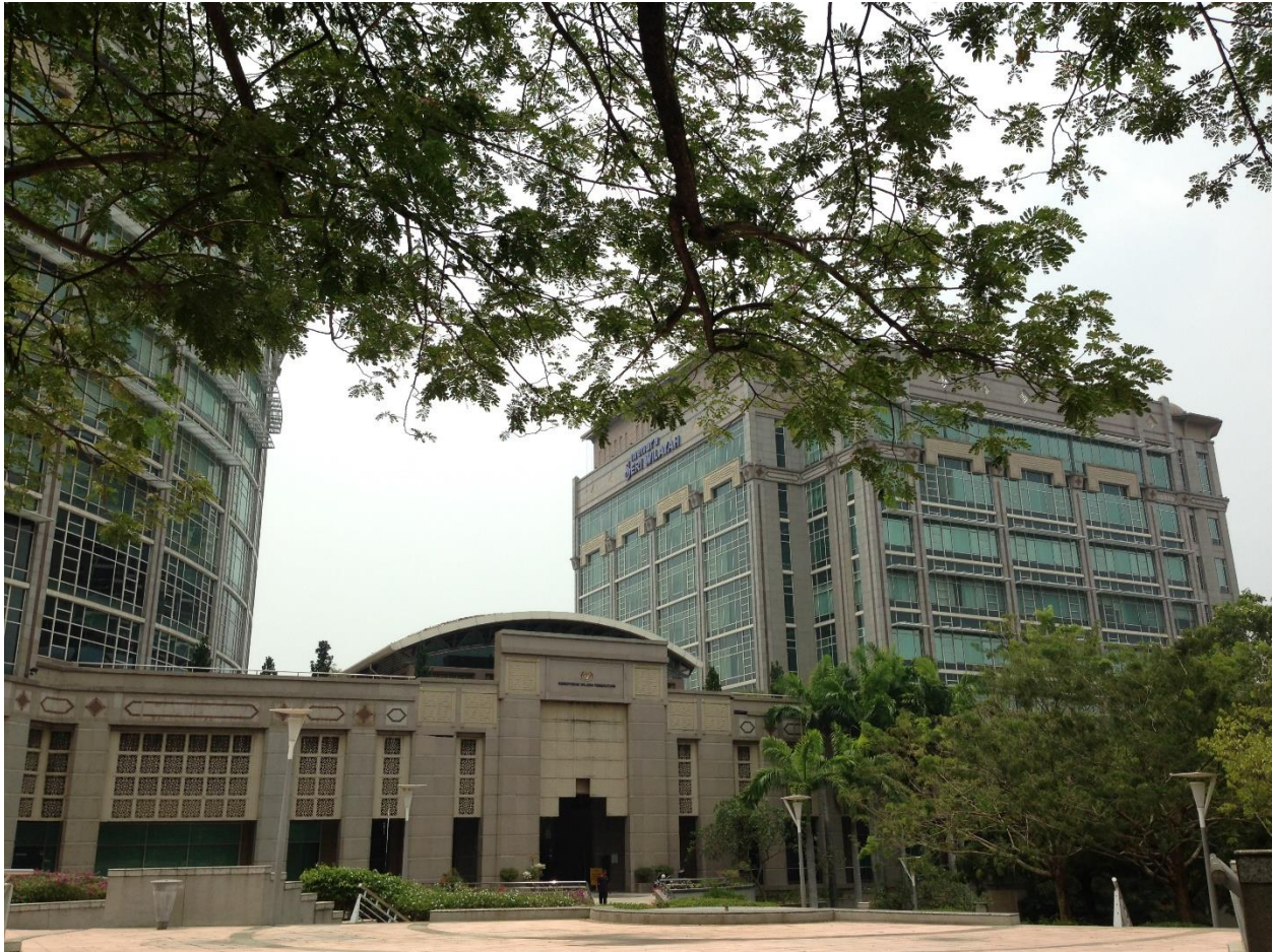
Figure 2: An image of the case study building taken during a field visit.
