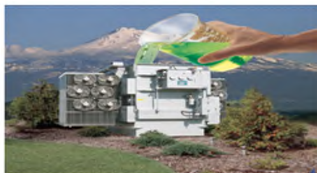
Fig. 1. Filling a transformer with envirotemp FR3 [5].
