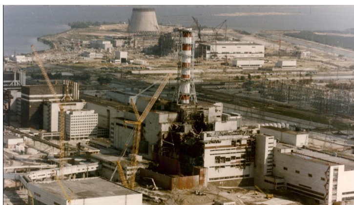
Figure 1: Aerial image of the Chernobyl nuclear power plant after the explosion of Unit 4 (BBC).
