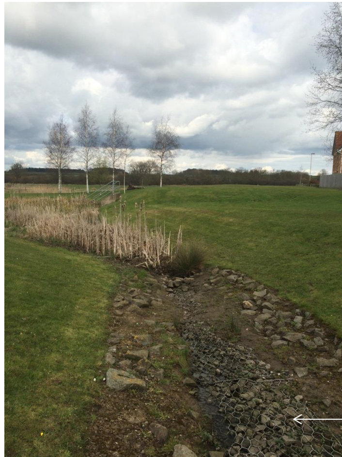
Figure 3-31 Site 8: Measurements were taken before the rip-rap at the end of the central swale train.
