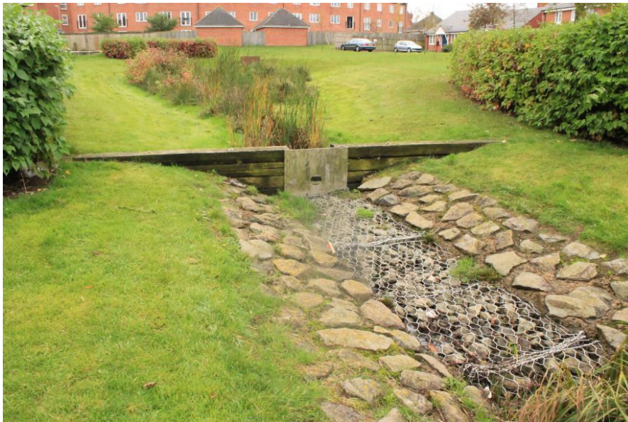
Figure 2-17 Weir at the SuDS management train in Hamilton, Leicester that causes runoff to backfill through the system, utilising vegetated ponds to manage flood events.
