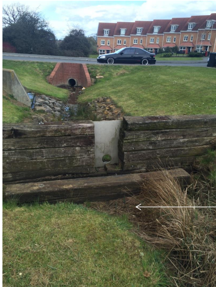
Figure 3-26 Site 3: Measurement was taken before the weir.
