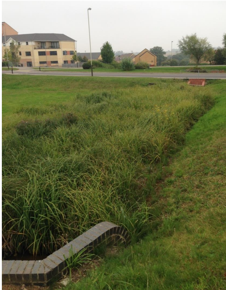
Figure 3-20 Vegetation filled pond 1, a densely vegetated pond with the offline detention basin to the left of the picture.
