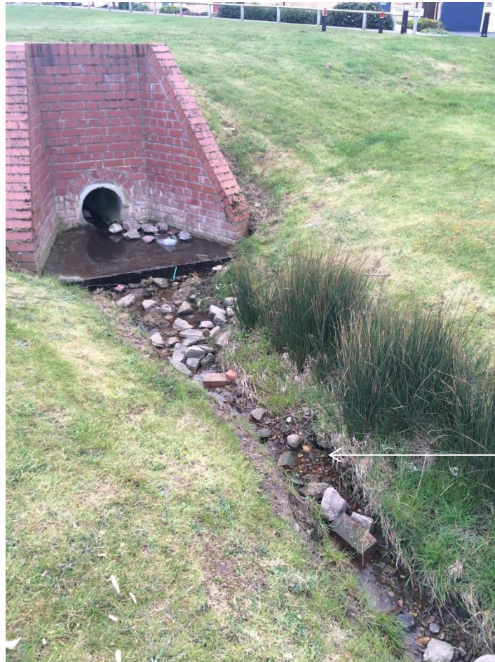
Figure 3-27 Site 4: Measurements were taken at the start of the narrower ditch. Debris from surrounding building sites was typically present at the site.
