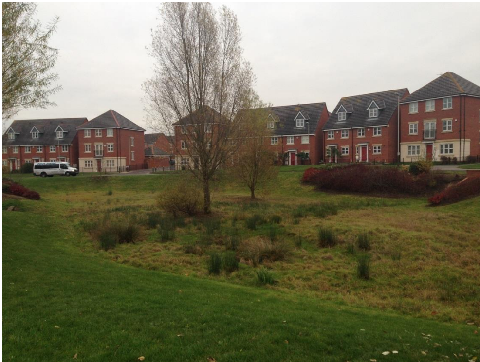
Figure 3-21 Detention basin 2: a large open pond that is densely vegetated. A small channel runs through the detention basin to direct runoff through the system.
