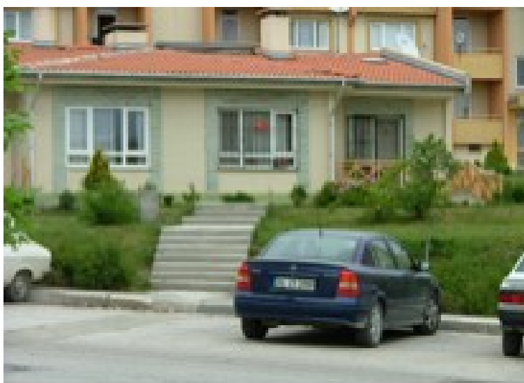
Figure 5.13: Steep stairs leading to houses designed for disabled and elderly people.
