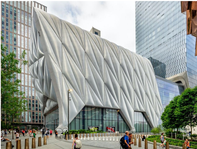
Figure 3 Moveable telescoping roof of The Shed, New York (Photograph by Ajay Suresh)
