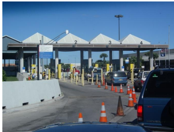
Fig. 1. Land border crossing with several lanes and a portal monitor in each lane.
