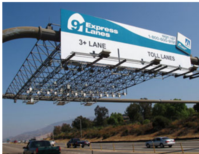
Figure 2. SR-91 Lane Designation Overhead Sign (OCTA 2009)
