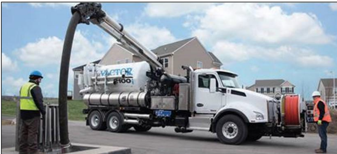
Vacuum trucks remove sediment from a catch basin.
