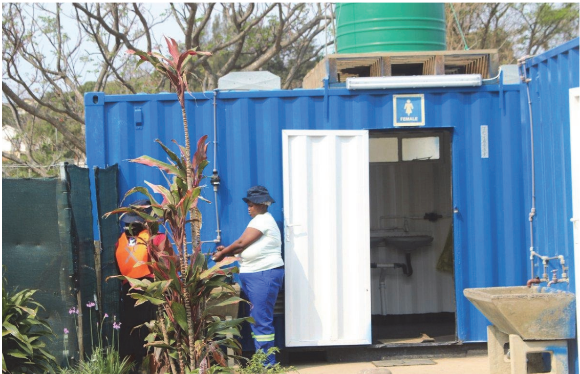
Figure 2.7 Community ablution blocks in Durban, South Africa (source eThekweni Municipality, photo: UKZN PRG).
