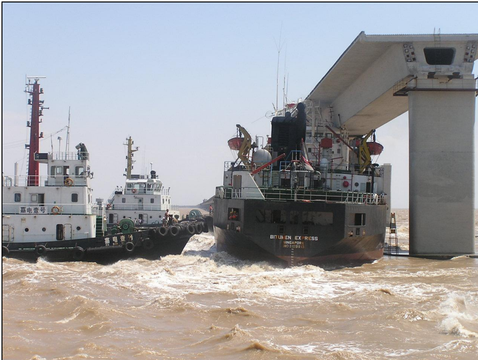
Figure-7 Accident photo-1
