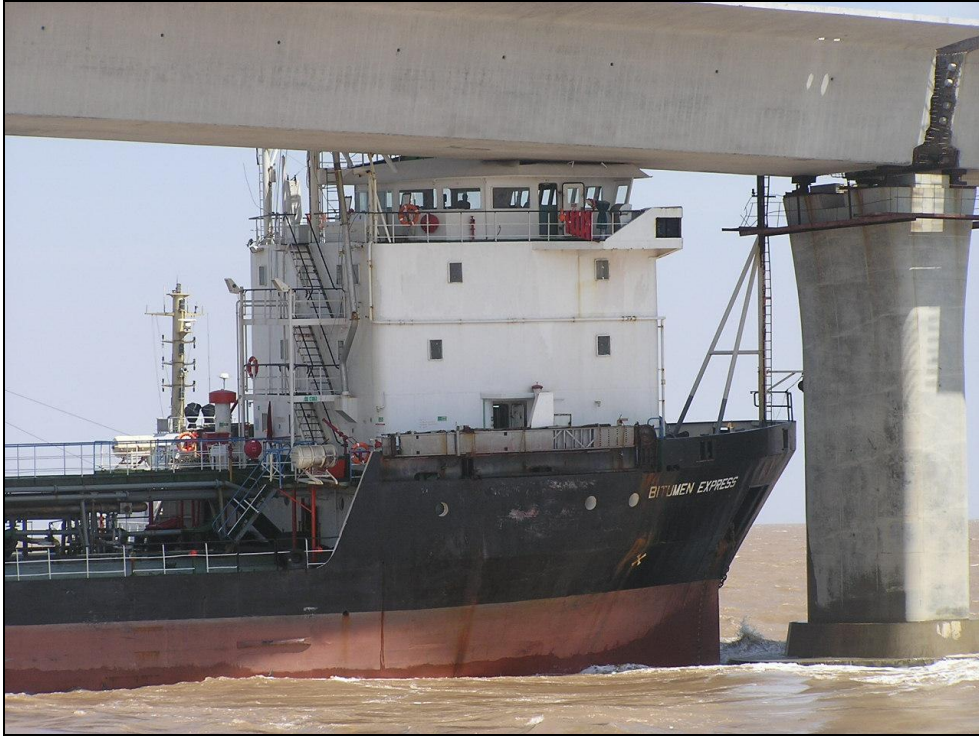
Figure-8 Accident photo-2
