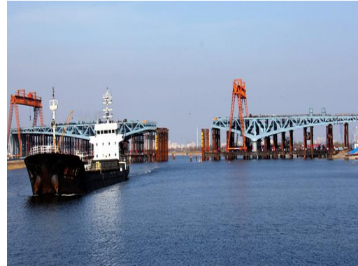
Figure 3.2.5(2) West Outer Ring Bridge
