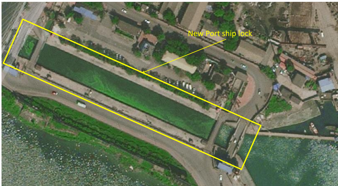
Figure 3.2.4 (1) New Port ship lock
