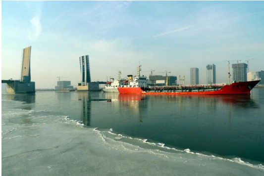
Figure 3.2.4(3) Haihe open bridge
