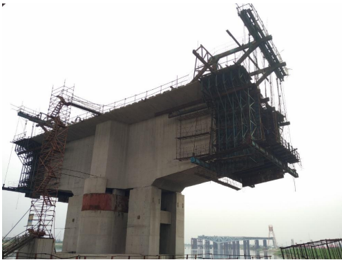
Figure 3.2.5(1) Binhai Bridge Extension
