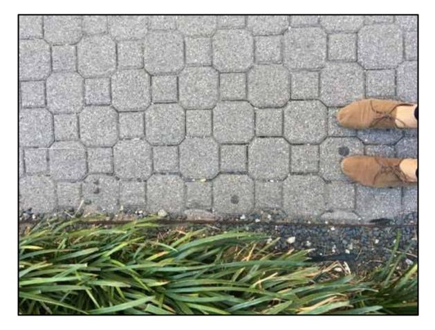
Figure 12. Permeable Pavement in Dallas, Texas<sup>165</sup>
