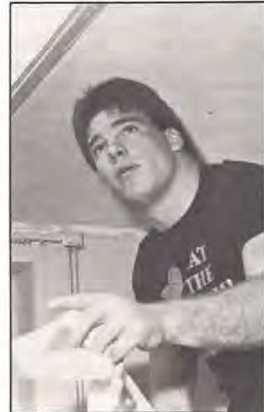
■ A Red Shirt member repairs a ceiling.
