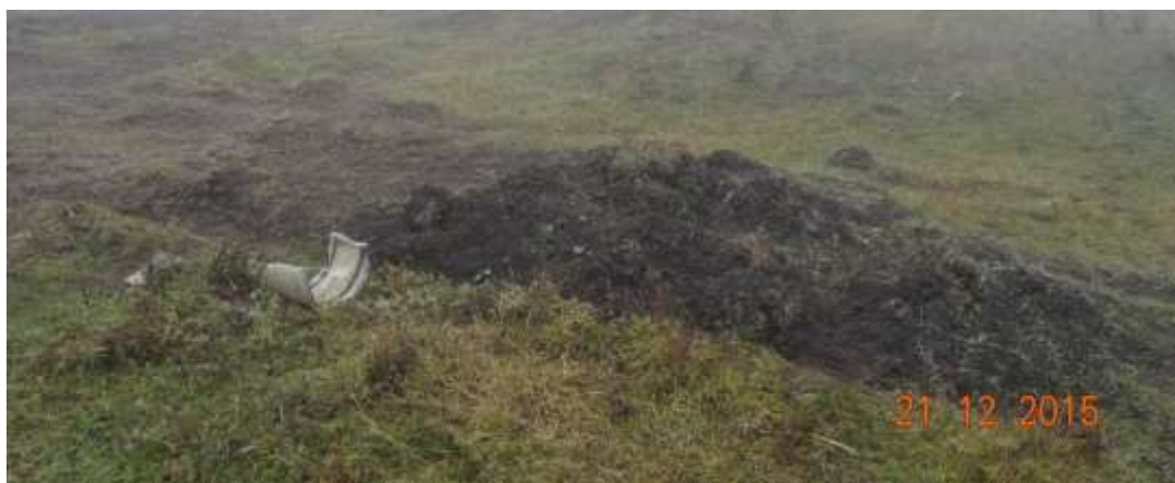
Figure 3 Detail on the state of pipe sections made of asbestos tubes (damage to joints, tube breaks) (Luca M., 2016)
