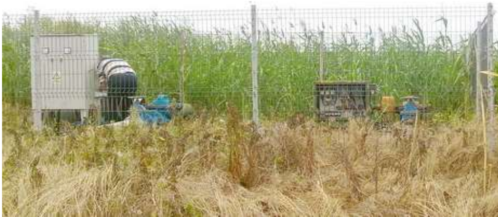
Figure 6 General view of Doniceasa-Fălcu Plot 7 SPPM 7/5 partially rehabilitated (replacement of an electric motor and the electric panel for the pumping unit 7/5-1) (Photo Luca M., 2016)
