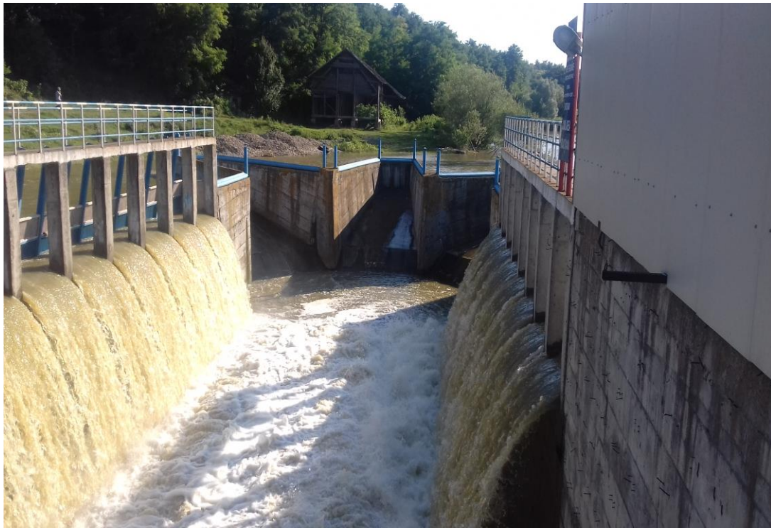
Figure 5 Dracsani dam – discharge over the surface spillway
