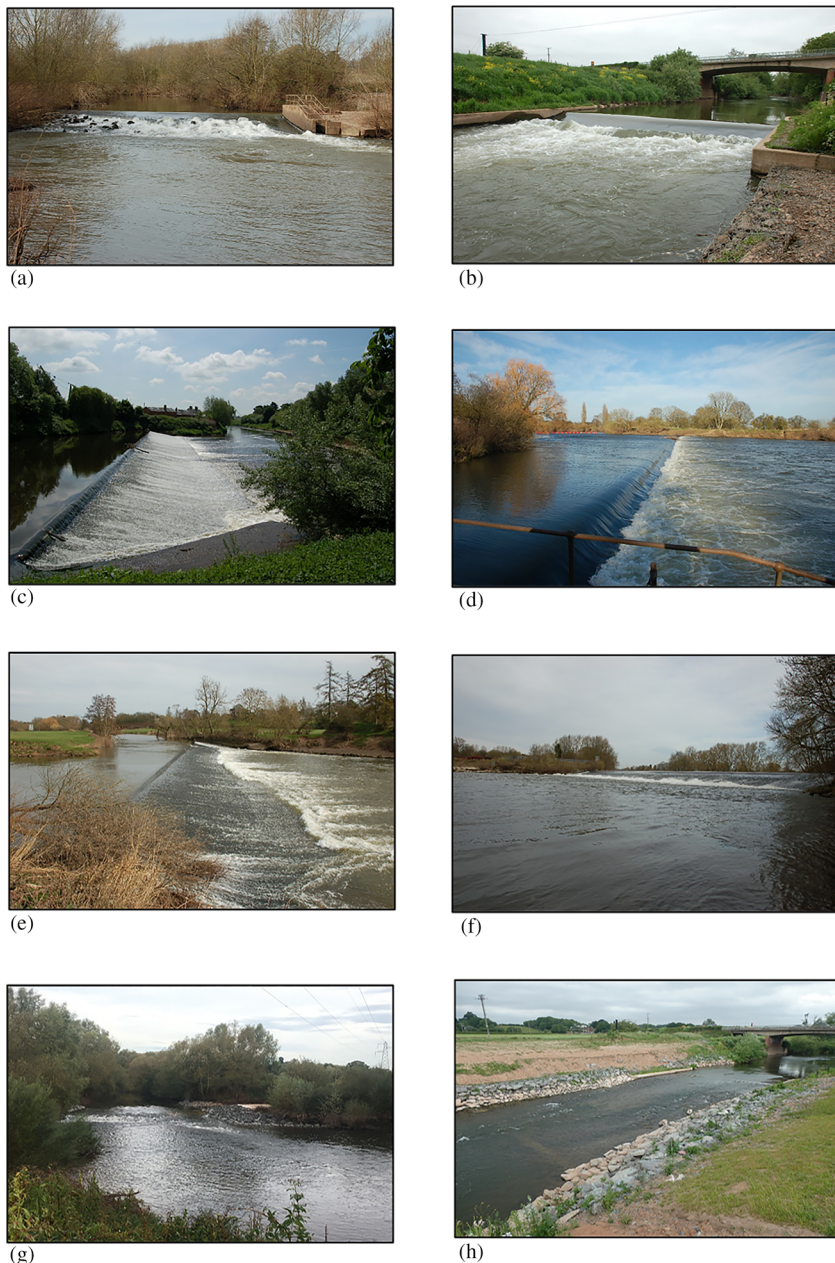
FIGURE 2 (a) Powick Weir prior to modifications during sampling in 2017 and 2018, and considered as largely impassable to shad. (b) Knightwick Weir prior to modifications, during sampling in 2017 and 2018, considered an obstacle to migrating shad. (c) Diglis Weir, considered to be impassable to shad. (d) Upper Lode Weir, in the lower reach of the River Severn, considered not to be a major obstacle to fish migration. (e) Bevere Weir, an obstacle to migrating shad on the River Severn. (f) Lincomb Weir, an obstacle to migrating shad on the River Severn. (g) Powick Weir following weir modifications in 2019. (h) Knightwick Weir following modifications in 2019
