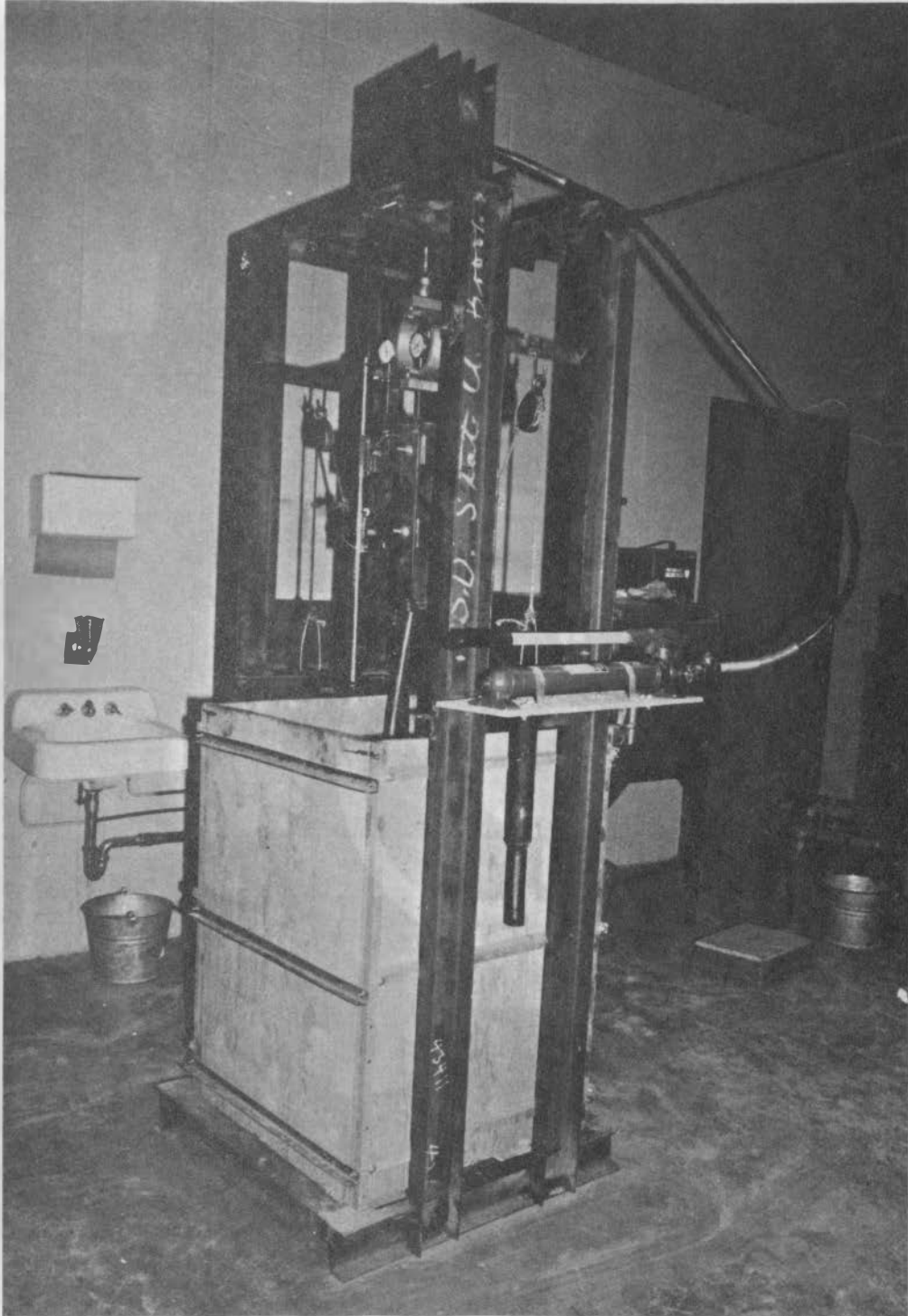
FIGURE 10. PILE LOADING APPARATUS
