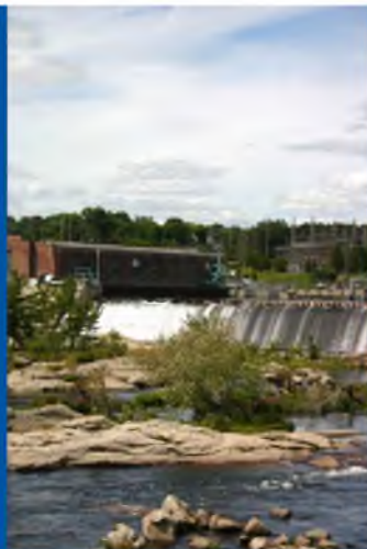
Amoskeag Hydro station, one of two hydro facilities in the City providing clean alternative energy
