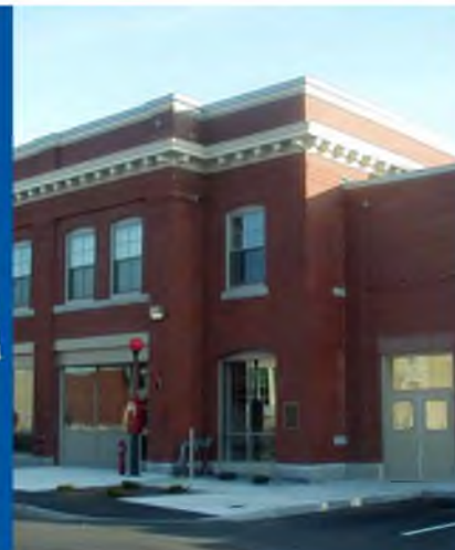
The renovated Station 7 on Somerville Street includes a new addition
