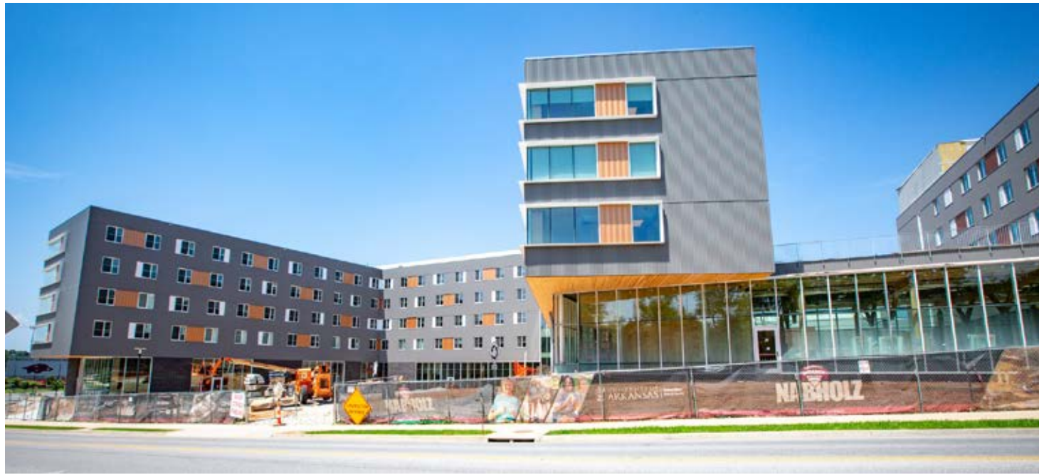
Adohi Hall, shown during construction in June 2019, on the University of Arkansas campus. (Photo by Whit Pruitt)
