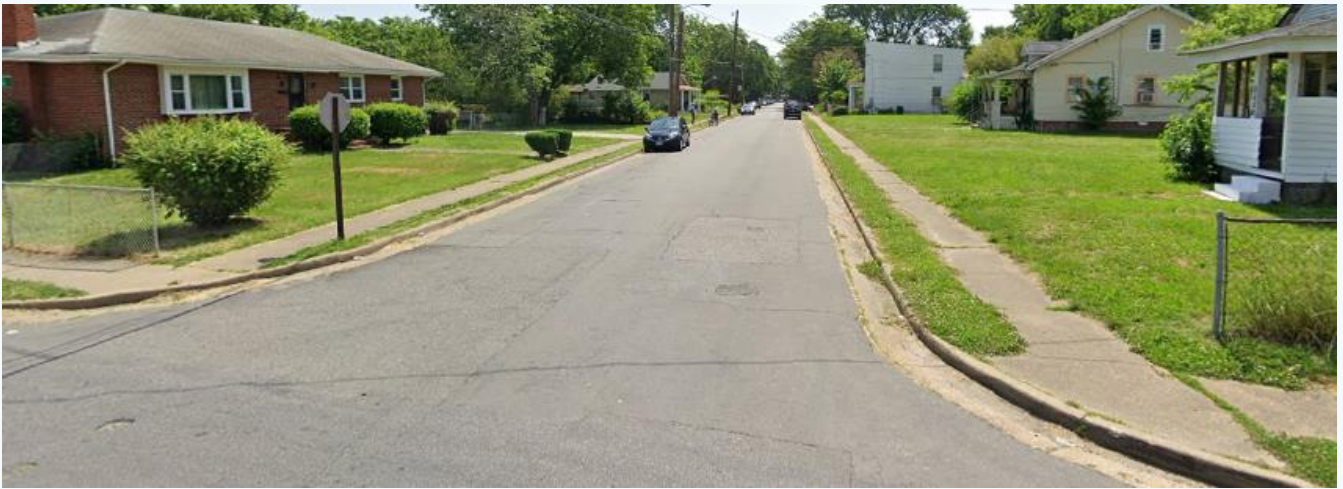
Figure 24. Inaccessible Sidewalk and Unsafe Crossing Areas; Source: Google Maps, 2019
