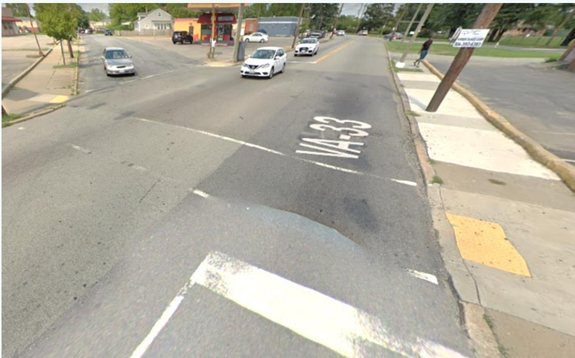
Figure 21. Intersection with Faded Crosswalk Paint; Source: Google Maps, 2019
