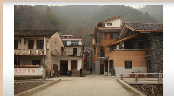
文村老村口改造后 The old entrance of Wencun village after renovation
