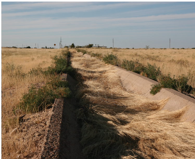
Irrigation Ditch near Pecos, Texas
