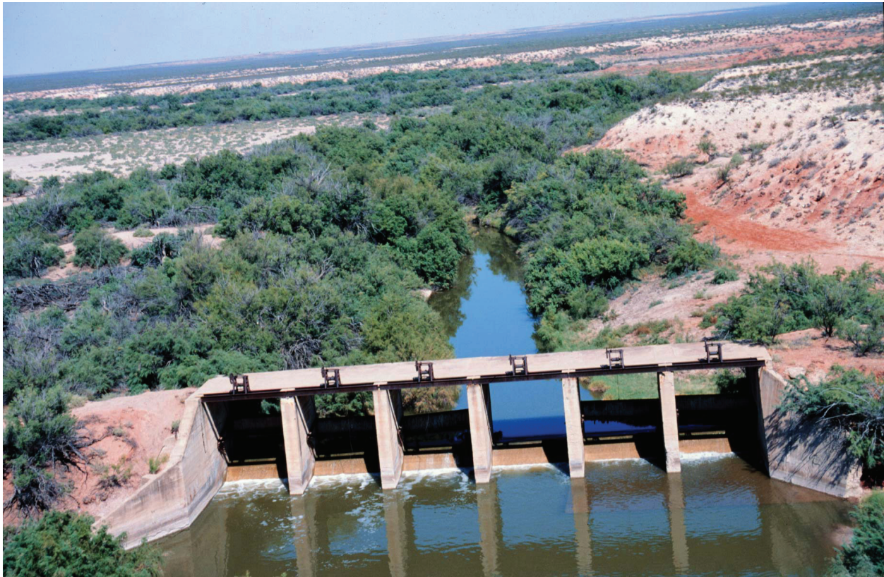
Irrigation diversion dam on the Pecos River near Coyanosa, Texas
