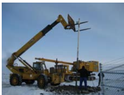
Lowering the 250-pound thermopile into position.
