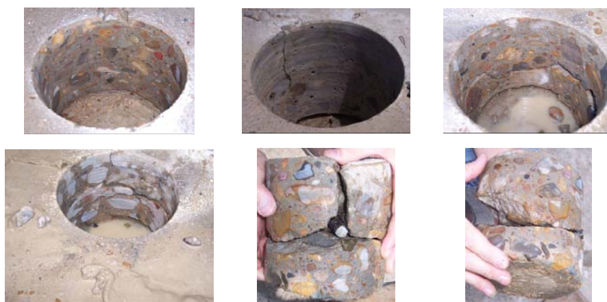
Figure 3-30 Interface and PCC Layer Condition of Section on IH 10.
