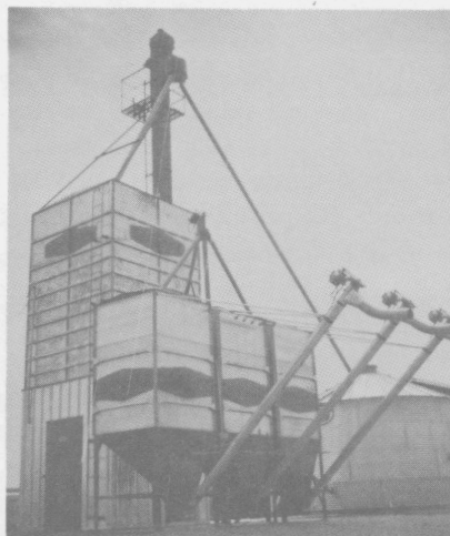
Figure 21. An automatic feed factory with three different ration bins for a swine operation.
