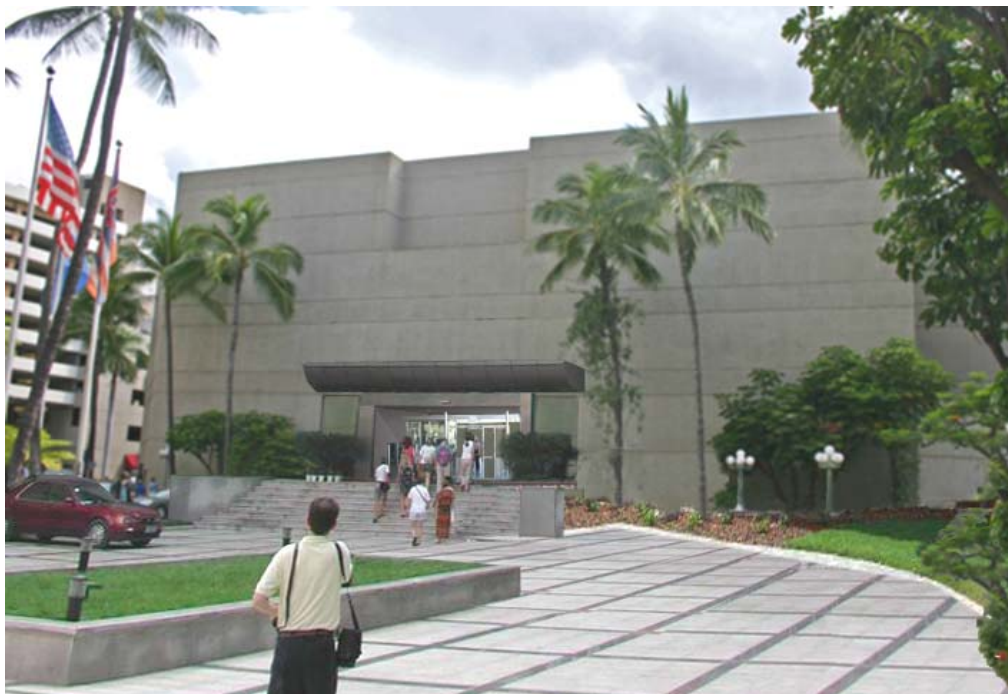
FIGURE 4.8. Study 3: Distant view of the building, depicting solid façade and access-control security measures that appear as part of the overall architectural design of the entrance.
