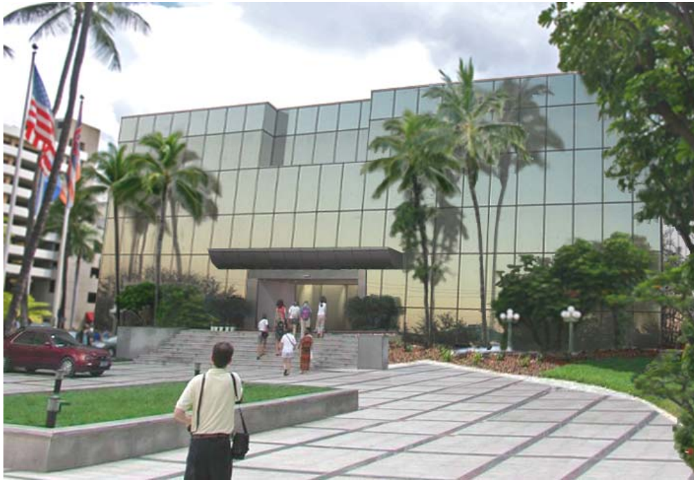
FIGURE 4.2. Study 2: Distant view of the building, depicting an all-glass façade.
