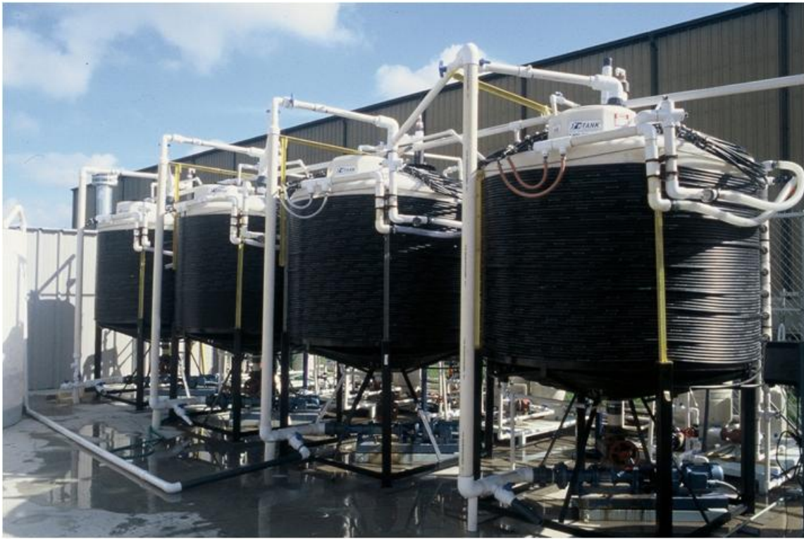
Figure 7-1. Photograph of countercurrent fermentation reactors in pilot plant (College Station, TX).
