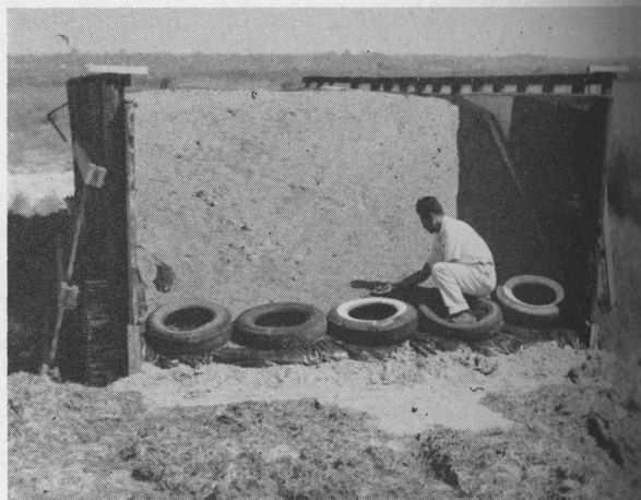
Figure 2. Temporary sideboards were helpful in forming stack silos. Posts were set loosely in slightly oversized holes (top). Posts and walls were removed after the stack was completed (bottom).
