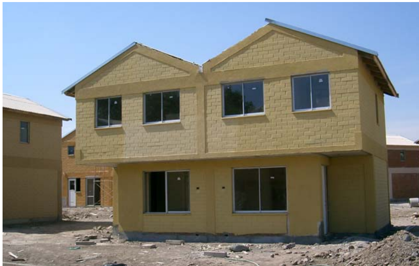
Fig. 3. Confined masonry house near completion
