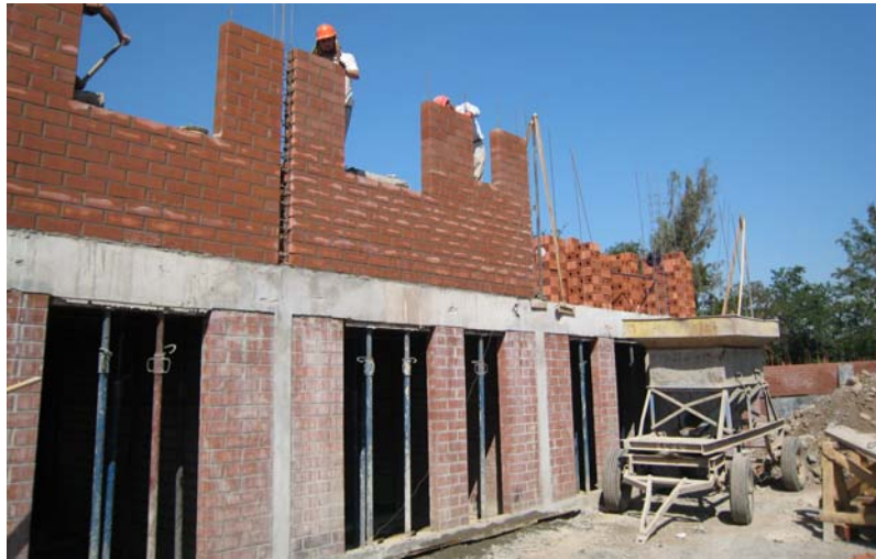
Fig. 2. Confined masonry construction in Maipú, Chile
