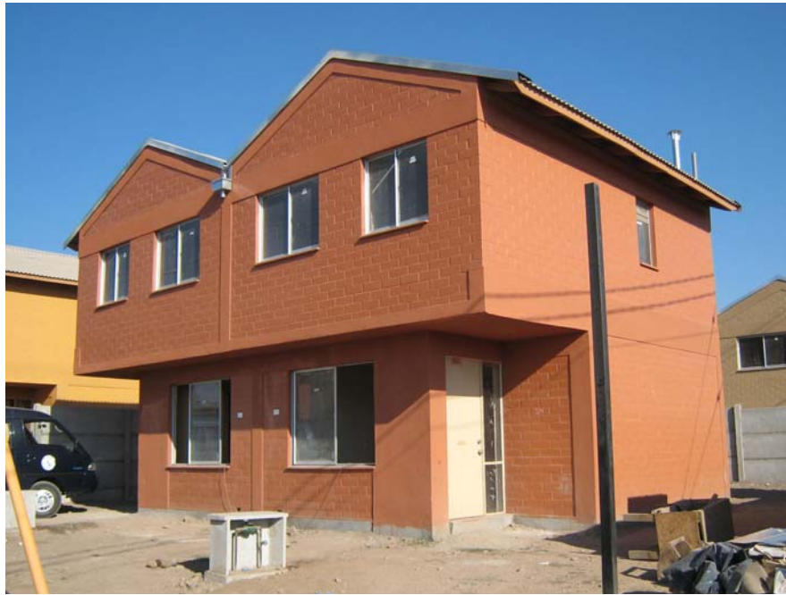
Fig. 22. Front view of test structure
