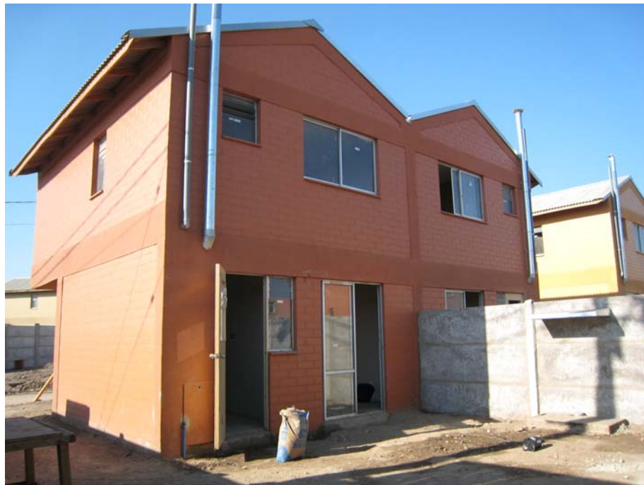
Fig. 23. Back view of test structure
