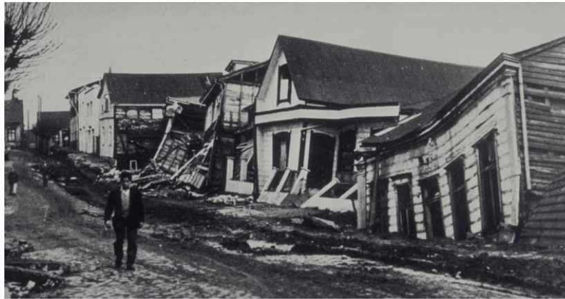
Fig. 1. Damaged houses after 1960 Chile earthquake ( www.ngdc.noaa.gov )
